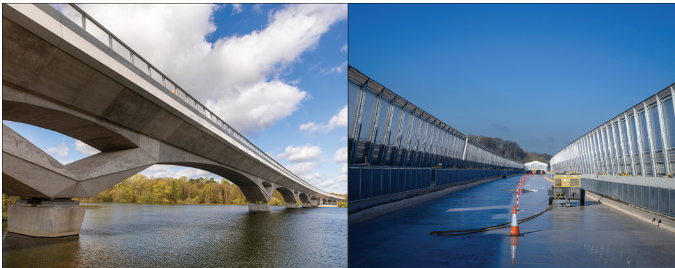
Transparent noise panels and absorption panels on the Colne Valley Viaduct, part of the new HS2 line © HS2
