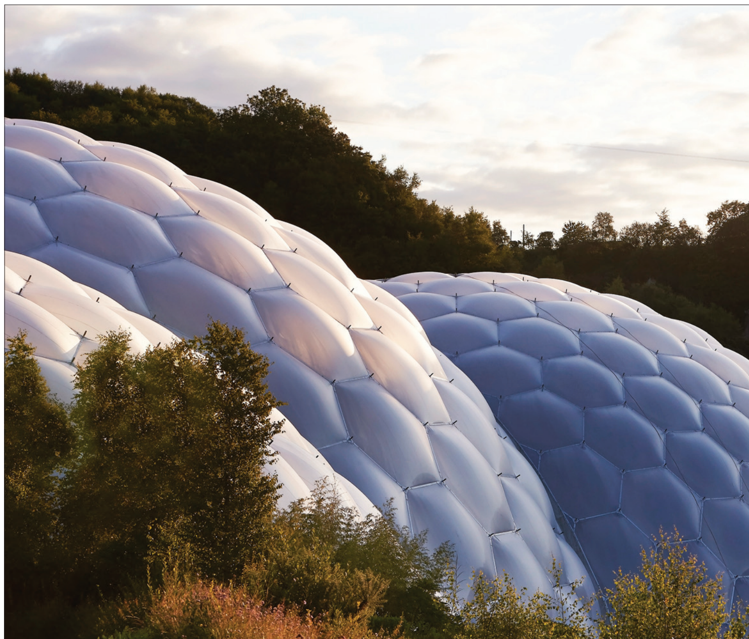
The Eden Project in Cornwall heats its biomes with geothermal energy, thanks to its spinout company Eden Geothermal © Hufton + Crow
