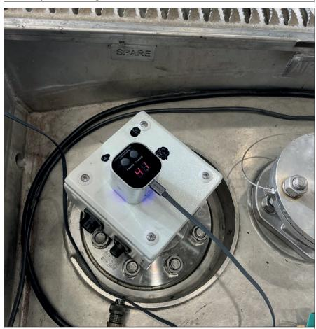
The sensor installed at the top of liquid storage tanks. Installing the sensors in hard-to-reach areas such as these is particularly beneficial. Condensation can form at the top of storage tanks, which could promote more bacterial growth that may otherwise not be detected © Phil Marsden
