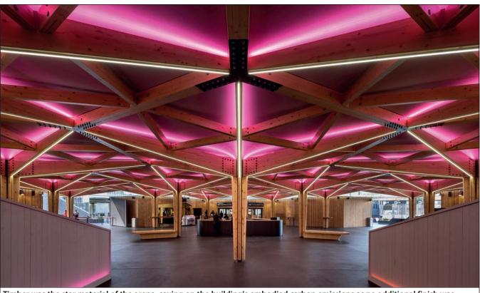
Timber was the star material of the arena, saving on the building's embodied carbon emissions as no additional finish was needed © Dirk Lindner, Stufish
