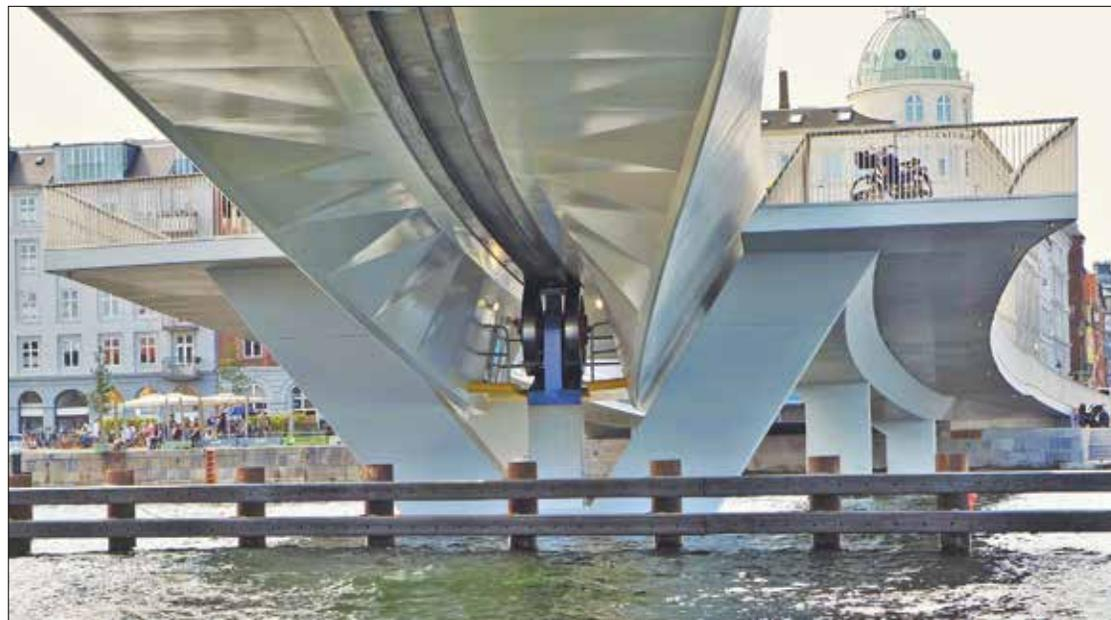
The underside of the bridge shows where the inner webs were divided into triangles. This gives an interesting crystalline appearance when viewed from the underside as the light reflects off the water. The fixed forward rollers and the transverse guide wheel are just visible. The guide wheel runs along a slot to control the extending position of the moving spans © Cezary Bednarski
