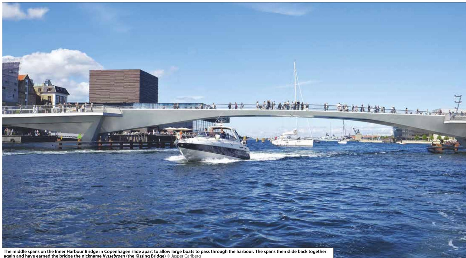
The middle spans on the Inner Harbour Bridge in Copenhagen slide apart to allow large boats to pass through the harbour. The spans then slide back together again and have earned the bridge the nickname *Kyssebroen* (the Kissing Bridge) © Jasper Carlberg
