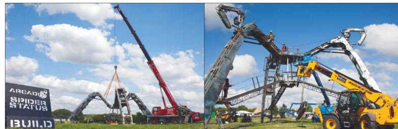
After the legs are attached to the Spider's main body, a crane lifts them up so that they pivot and stabilise the structure (left). Ancillary components are attached using hydraulic platforms (right) © Giles Mayall
