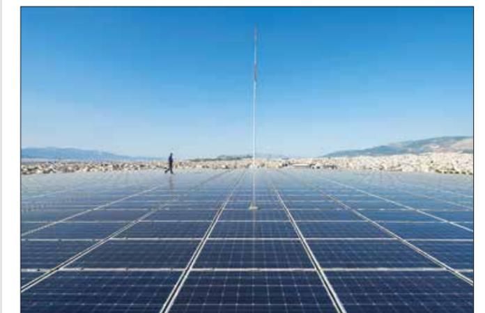
The tight packing of PV cells on top of the canopy was achieved by laminating the panels so that they can be walked on, which removes the need for maintenance walkways © Michel Denancé
