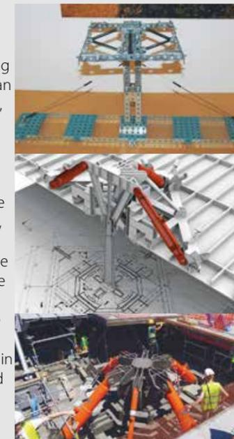
The column-head springs to support the canopy: an early Meccano model to test the concept (top); a 3D model to aid construction (middle); and a completed column head in place (bottom) before installing the ferrocement panels over the top. The large orange elements are the fluid polymer springs © Expedition Engineering
