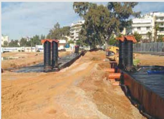
**Onsite surface water attenuation is provided throughout the park in the form of geocellular tanks and deep gravel trenches. Both act to store water during times of heavy rainfall, which protects the municipal drainage system from being overloaded and allows for infiltration to recharge the aquifer** © Michel Denancé
