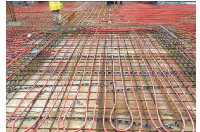
Red pipes that will carry chilled water for the concrete core cooling are laid over the mesh of reinforcing steel, before concrete is poured over both to create one of the floor slabs © Arup
